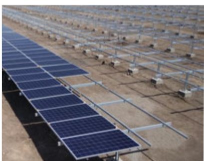
Solar Panel Structure Mounting on Ground
