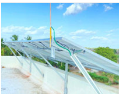
Solar Panel Structure Mounting on RCC
